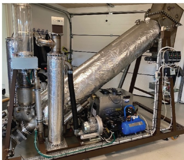
Almost finish plant in workshop - lacks control
