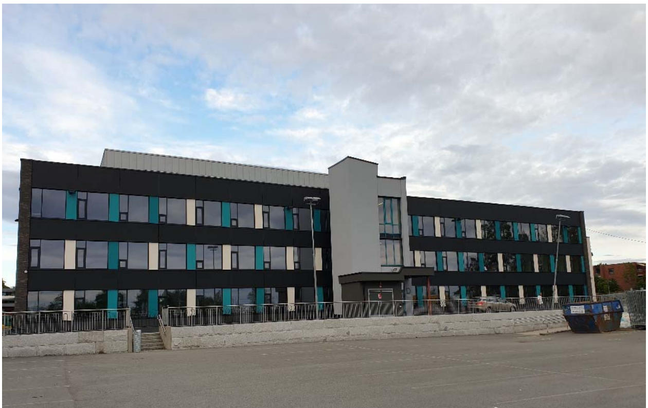
Figure 4.2(B).5 Cost-effective aesthetic rail-mounting final result.
