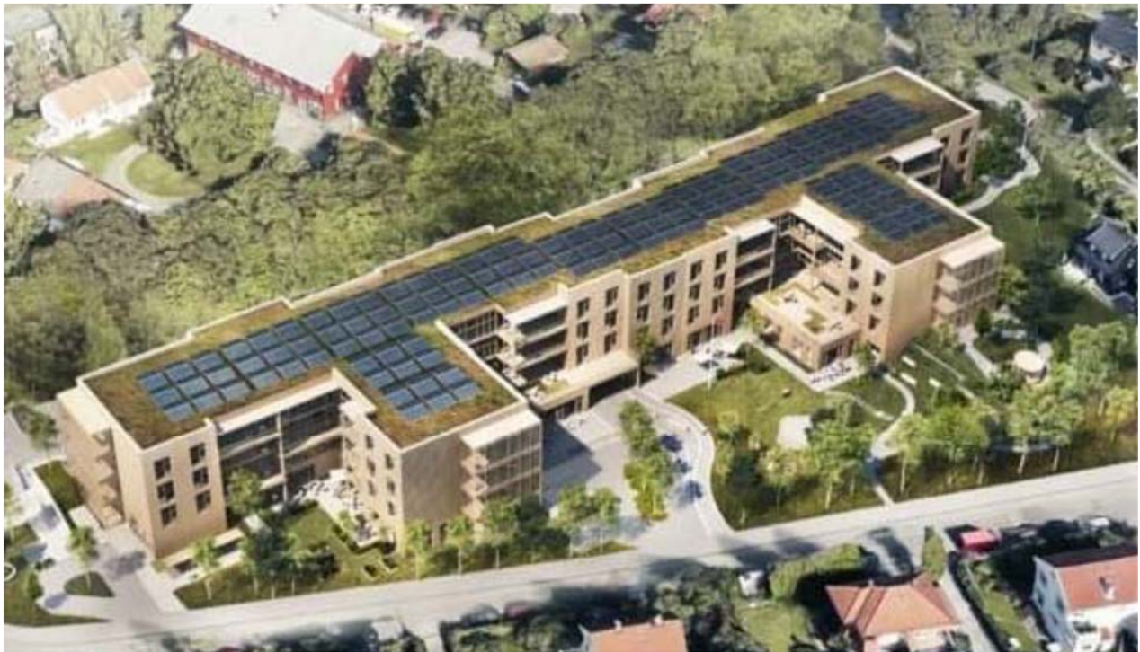
Figure 4.3.1.a Tåsenhjemmet in Norway, where simulations showed that Solar CHP-C could provide self sufficiency for covering all of the required energy consumption.
