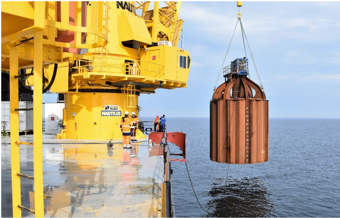
Figure 5 Preparing for suction at site B6
