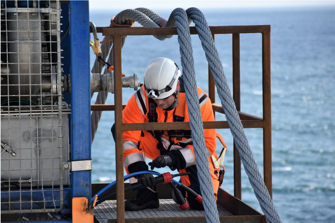
Figure 2 Connecting all the right cables to the pump unit
