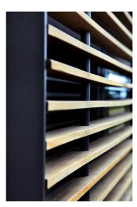
Solar shading from the inside and the outside. The frames are in aluminium, and the blinds are in mahogany wood. The prototypes were produced by Solatek, following a detailed design developed by IEN Consultants.
