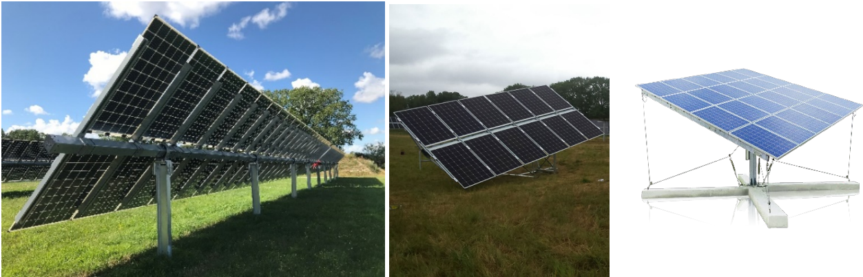
Figure 8 – different tracker configuration tested in the project. From left to right respectively the 1, 1.5 and 2 axis trackers are shown.
