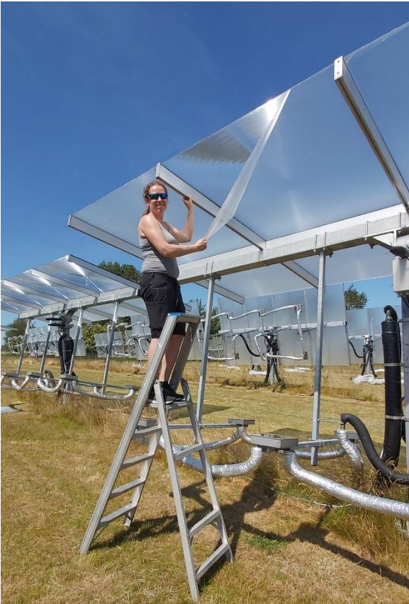
Casting film removal after lens installation (left) and the solar field after installation of new lenses (right).
