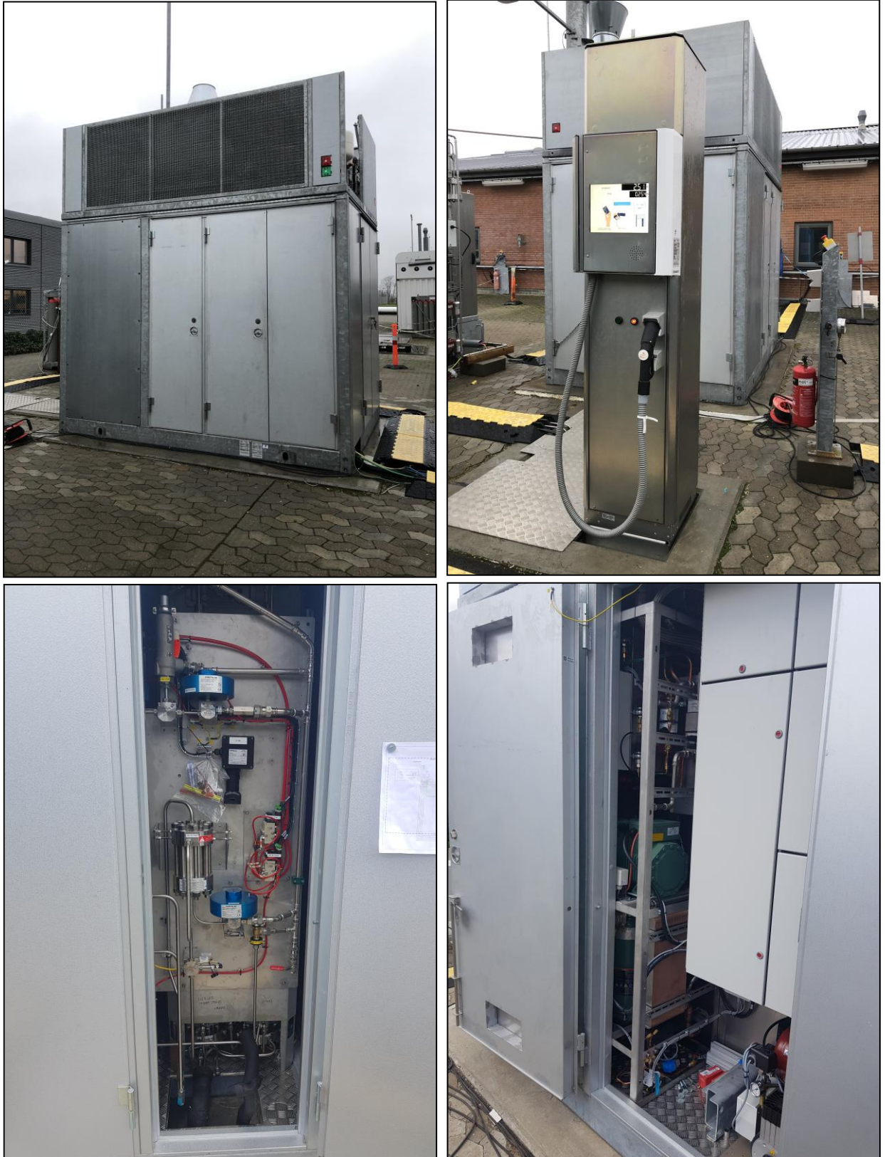
Figure 3.5.2.3 – Pictures of constructed cooling system prototype, integrated into H2Station®
