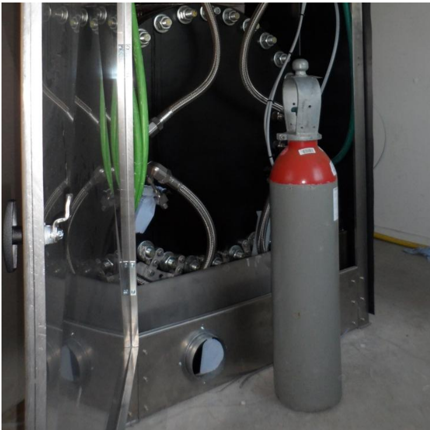
Figure 3: This cylinder was filled to 30 bars with hydrogen coming directly from the electrolyzer. Hereafter the cylinder was shipped to third party professional laboratory for detailed quality analysis
