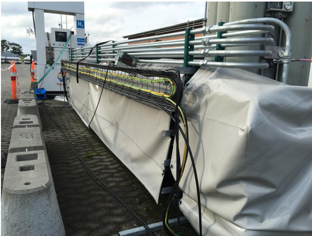
Figure 3.2.4.1 – Old dispenser pipeline design from H2Cost-1
