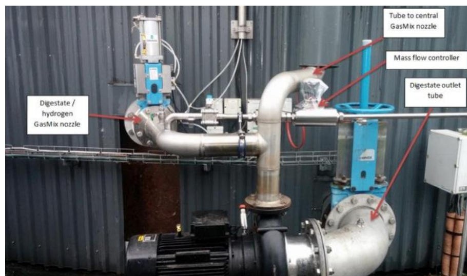
Figure 24 'GasMix' system for hydrogen injection to biogas reactors (Lan- dia A/S).
