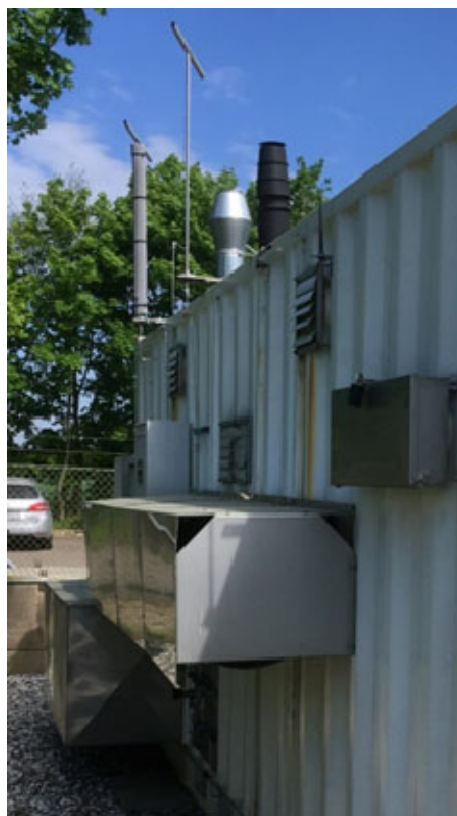
Figure 7. Hydrogen storage cylinder with protective cover.
