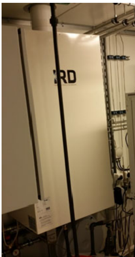
Figure 6. \mu\text{CHP} as wall installation.
