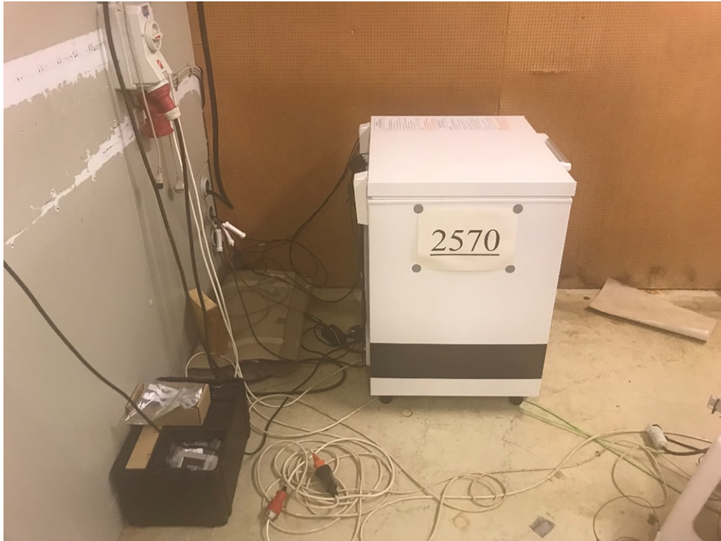
Figure 88 Mounting in climate chamber with high temperature and humidity.
