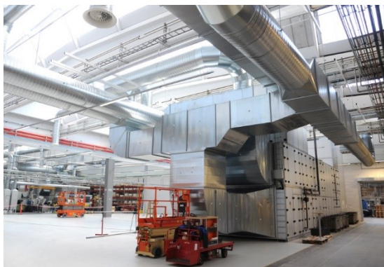
Figure 5. Left: large ventilation system installed in the production halls to collect exhaust heat from machinery. Right: Main ventilation system.
