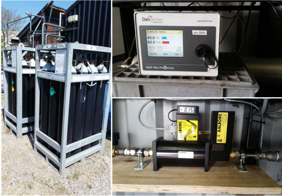
Figure 16 – Experimental setup for converting the air-blown gasifier to O 2 -CO 2 -blown. Left: Gas bottles. Upper right: gas mixer. Lower right: mass flow controller.
