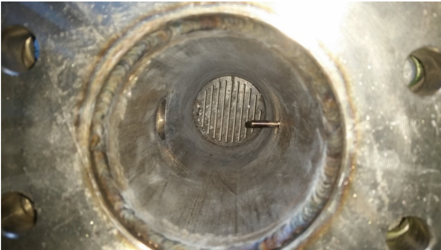
Figure 7 – Emptied and vacuum cleaned desulphurizer reactor
