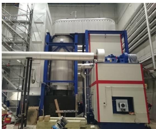
Wood chips and grain residues-fired boiler (KCO Kohlbach) with SNCR (ERC) (left) and electrostatic precipitator (Scheuch) (right) for process heat supply in the largest bakery in Switzerland. Photo by Verenum.
