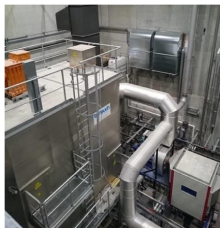
Wood chips and grain residues-fired boiler (KCO Kohlbach) with SNCR (ERC) (left) and electrostatic precipitator (Scheuch) (right) for process heat supply in the largest bakery in Switzerland. Photo by Verenum.
