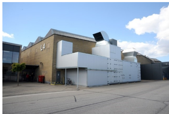
Figure 5. Left: large ventilation system installed in the production halls to collect exhaust heat from machinery. Right: Main ventilation system.
