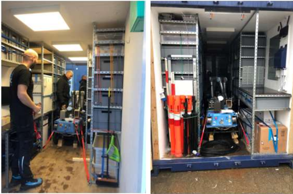
Figure 5 MRCC – from inside the rebuilt container
