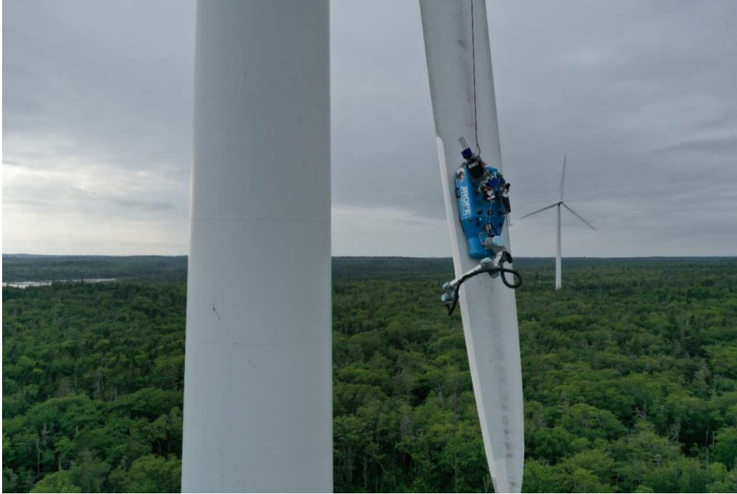
Figure 8 A complete leading edge repair done
