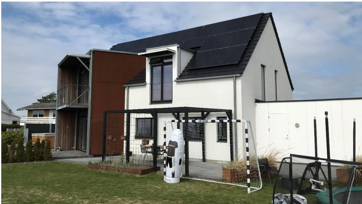
Figure 2 Test house in Kalundborg with existing PV system and heat pump.
