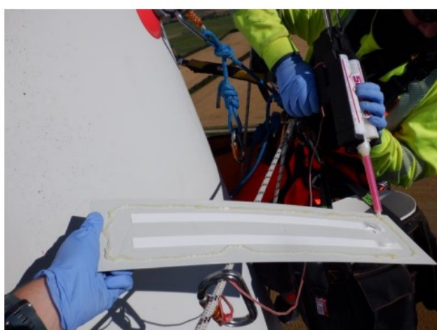
Figure 11: Installation of the standard PowerCurve SoA VGs to be used for comparison with the AdvancedVGs mounted on the neighbouring WT.
