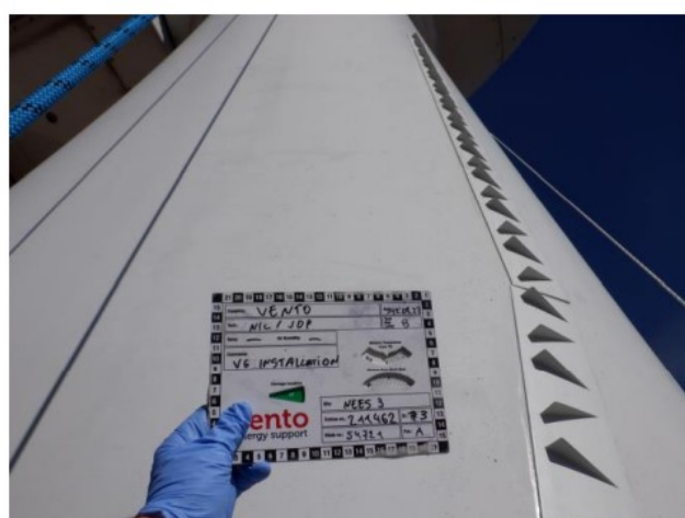
Figure 11: Installation of the standard PowerCurve SoA VGs to be used for comparison with the AdvancedVGs mounted on the neighbouring WT.
