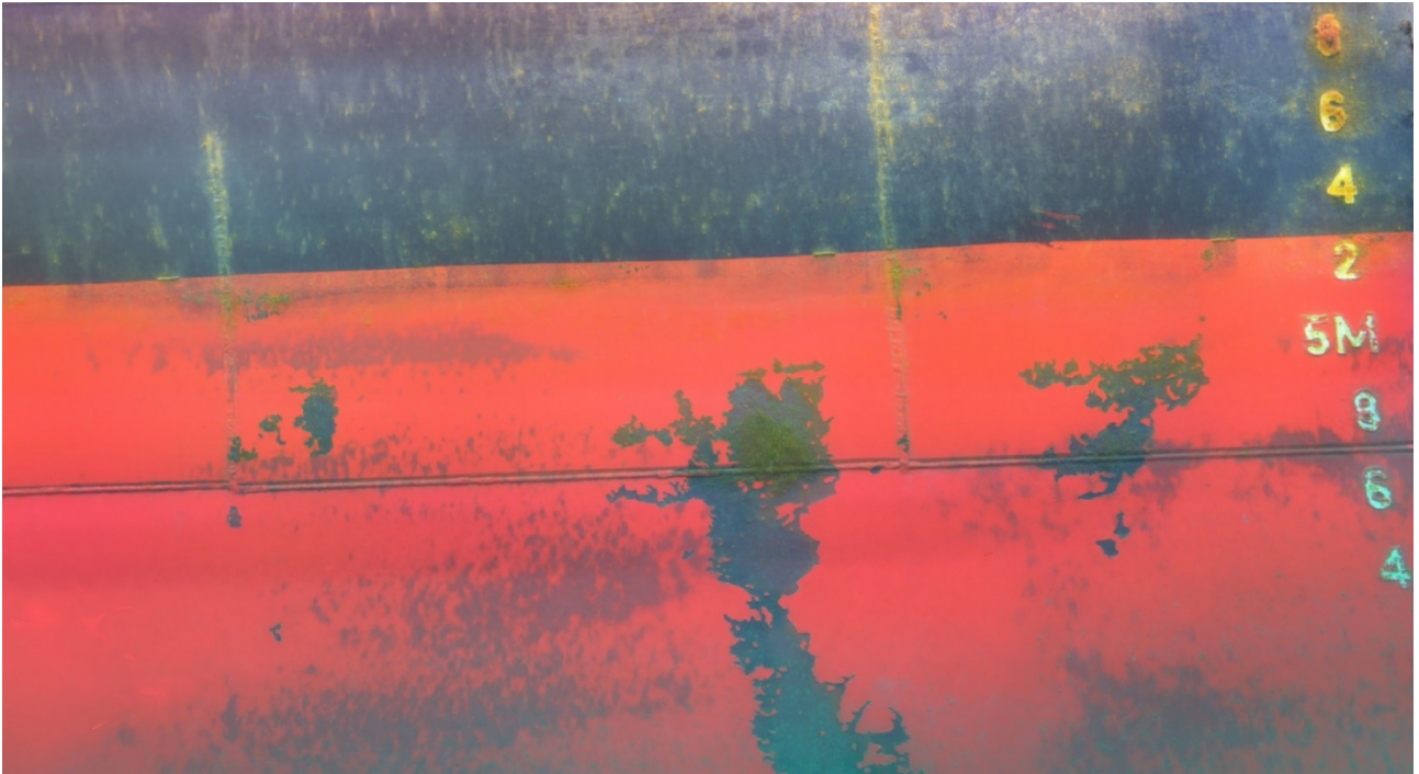
Figure 2 Example of 3D-model generated of side of a vessel, allowing for overview as well as detailed inspection of selected areas.
