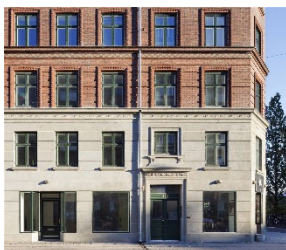
Figure 4. Ryesgade 30, before renovation.
