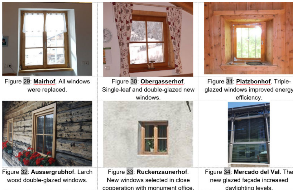
Figure 5. Examples of solutions where windows were replaced by handcrafted replicas.
