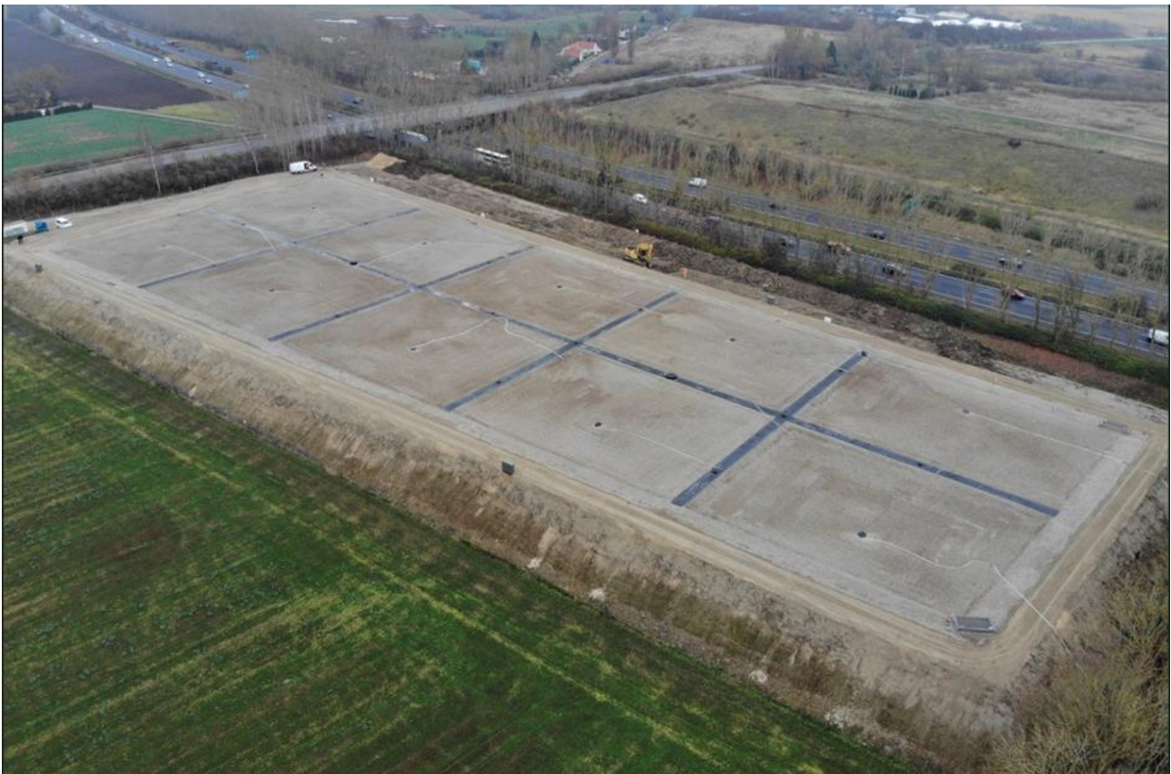
Aerial view of the 70'000 m 3 Pit Thermal Energy Storage owned by Høje Taastrup District Heating and VEKS Photo: Ioannis Sifnaios
