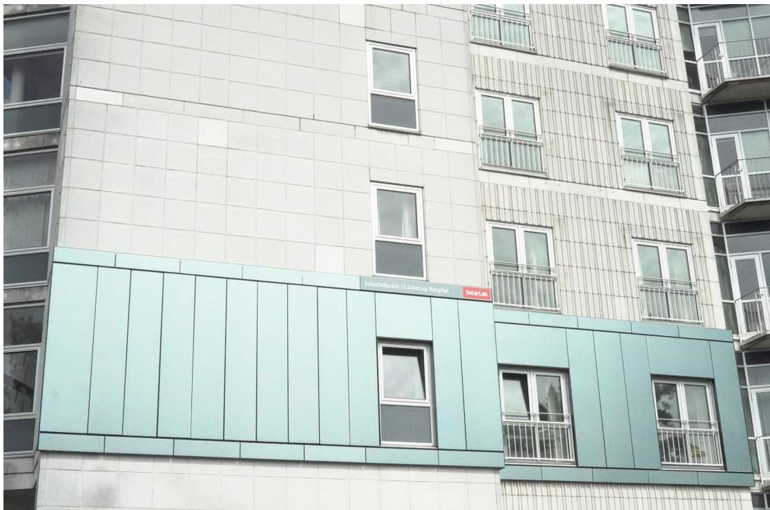
The hospital RH Glostrup: A SolarLab facade-mockup for a section of the building.
