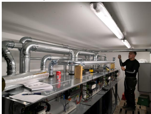
Construction of Nature Energy Nordfyn heat pump
