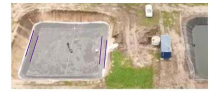
On the left is the completed bag, not yet covered with any overburden. (Colored lines are added to highlight the edges of the sloped region of the substrate.) On the right, a portion of the discharge reservoir is visible.
