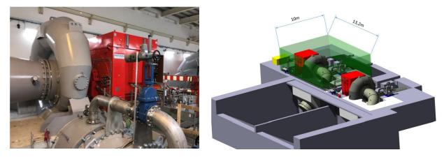
Fig. 4 The Turbine and generator of a hydro electrical system supplied by Voith and the corresponding physical outline.
