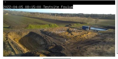
Photo taken the day before the bag rupture. In this photo, the orientation of sunlight and shadows is such as to make the overburden cracks (both peripheral cracks and straight-line diagonal cracks) especially visible. In this photo the bag was empty, as indicated by the fact that the water level is nearly full in the discharge reservoir in the rear of the photo.
