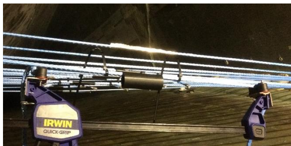
Figure 91 – Photo showing the rope tensioning and locking procedure
