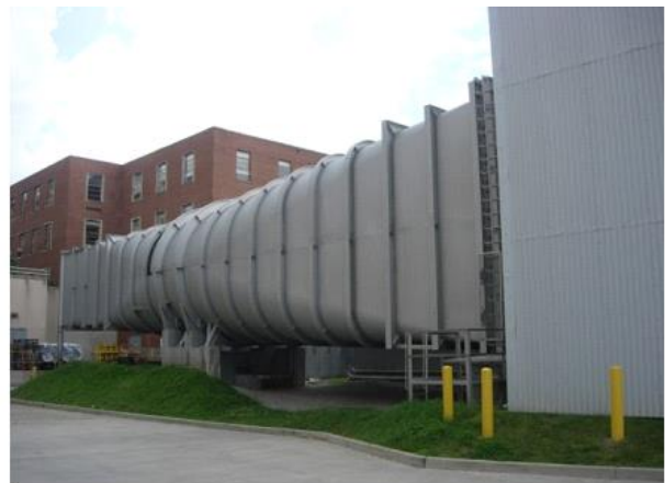
Figure 66 - Technological University of Virginia Wind Tunnel
