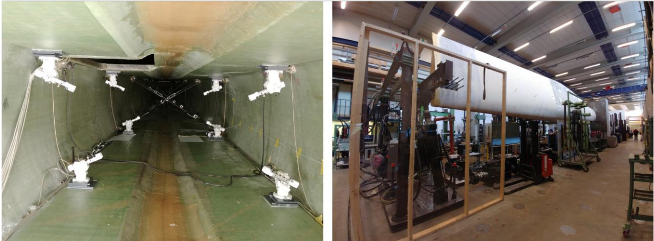
Figure 40 - CSSDS test integration at DTU, installed FCMs inside the blade (left) and test rig (right)
