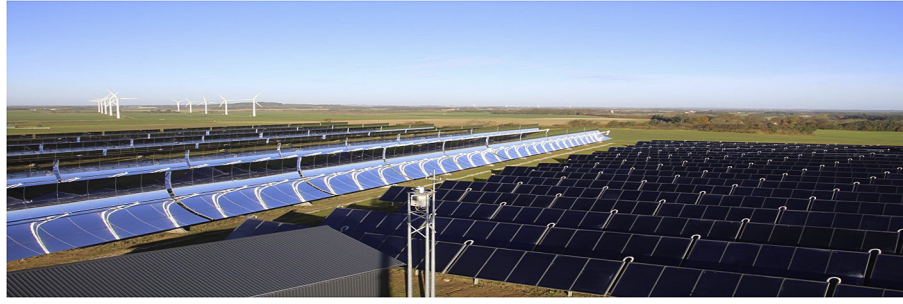
Fig. 1. Solar collector fields in the Taars solar heating plant [13].
