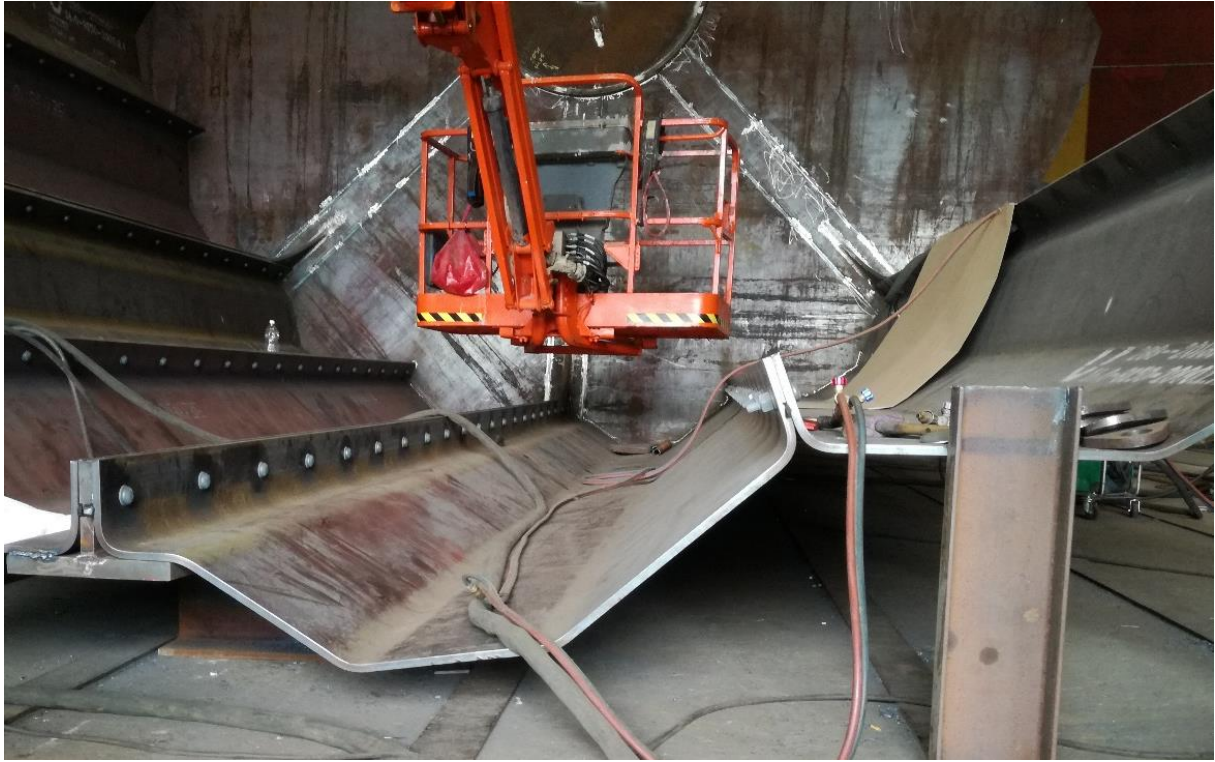
Figure 20 Assembly of the skirt sections
