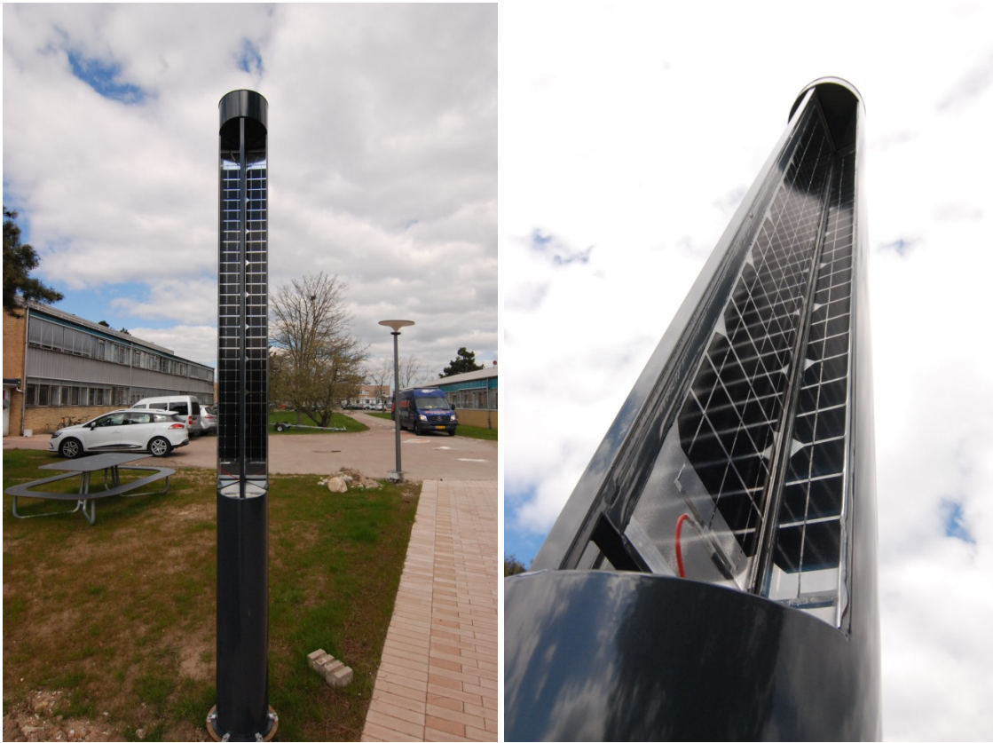
Figure 13: Photo of Sensorpower mast installed at DTU Fotonik in Roskilde.
