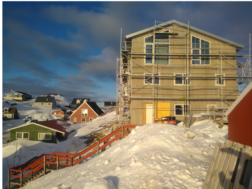
2017 Greenland Villa, 3 floors - 360 m 2 , Nuuk
