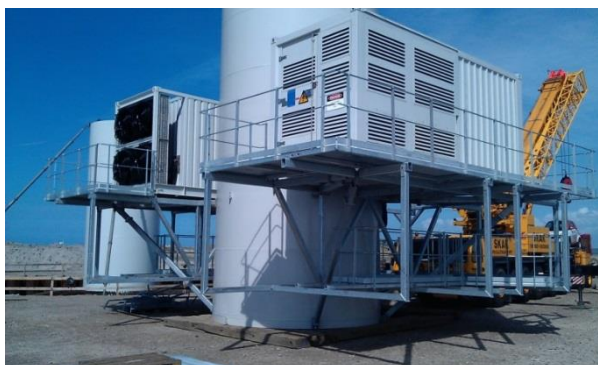
Figure 1 - GC1 - HV & Converter concept
