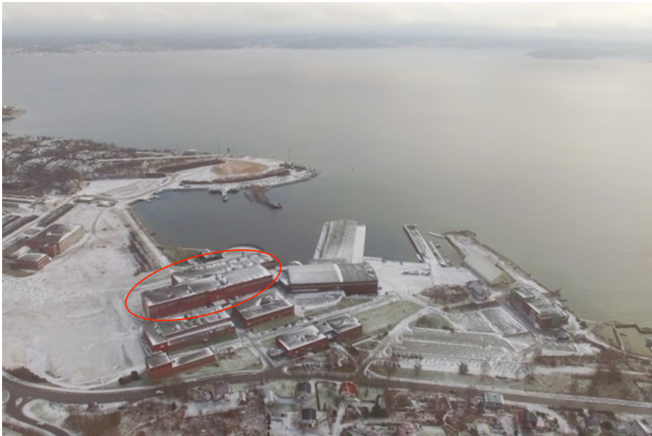
Figure 15: Silva Green Fuel project site in Tofte, Noway with existing building hosting the Industrial Demonstration plant.
