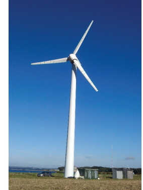
Figure 4. Vestas V27 wind turbine. The green strips on the blades are the tape protecting the accelerometer cables.
