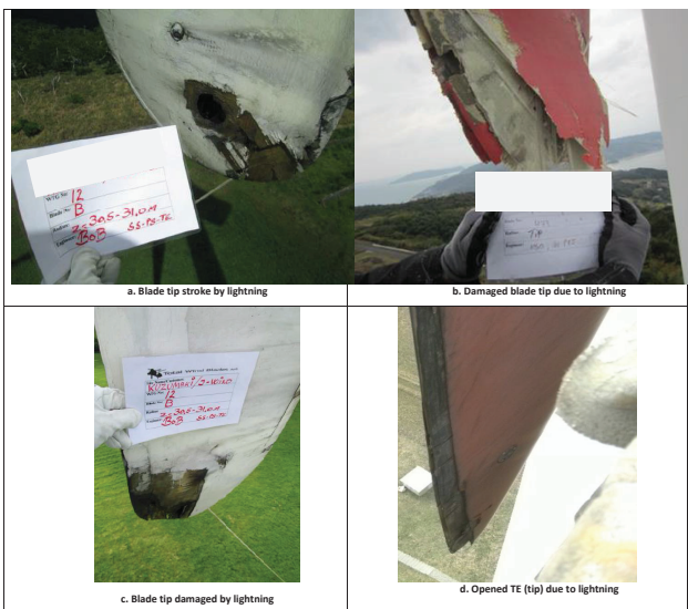
Figure 3: Blade damages caused by lightning strikes
