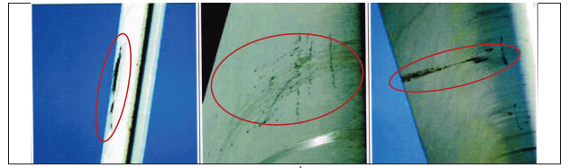
Figure 16: Bird impact: a. Impact produced a large crack in the panels; b. Damaged paint and first layer of the shell fiber; c. Small scratches in the shell
