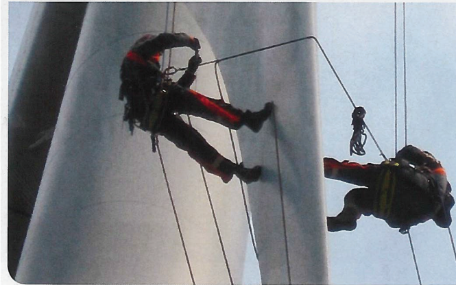
Technicians from Total Wind Blades ApS inspect a turbine blade.
