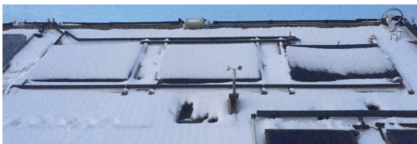
Figur 24. Snow partly melted on right PVT collector at 17:34 on 10/2/17.
