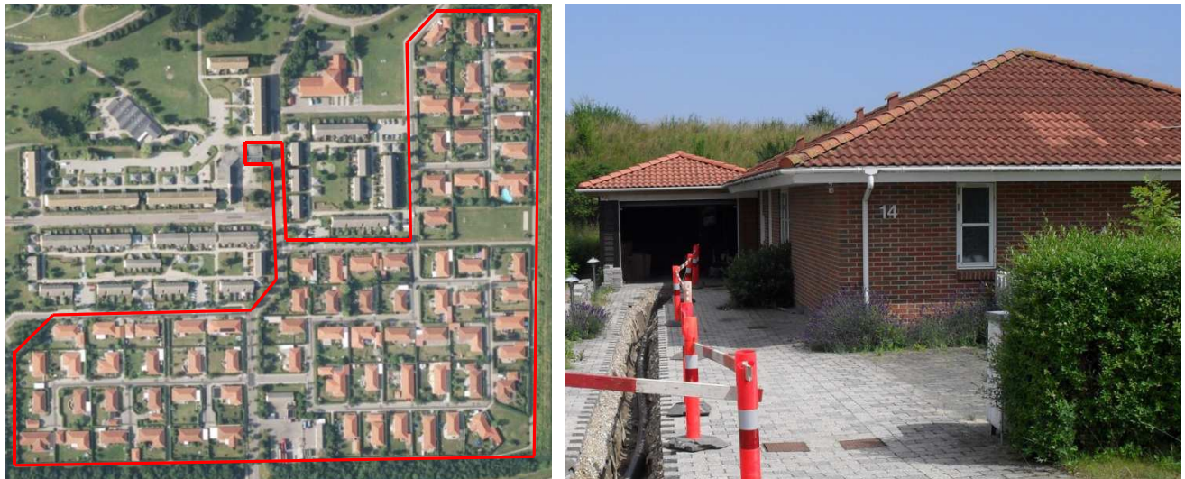
Figure A2.1 Air photo of the demonstration site area (marked with red) and an example of one of the 75 existing single-family houses, which got the new LTDH system installed.
