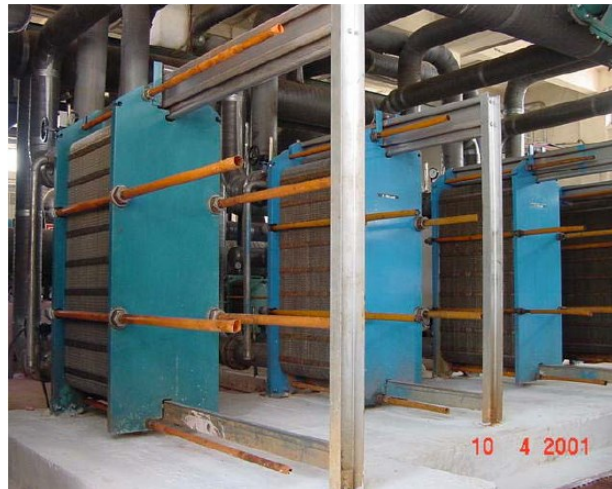
Figure 7 The plate heat exchangers used at Kırşehir DH system [1].
