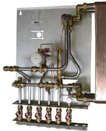
Figure 4.1 Picture of a low-temperature IHEU
