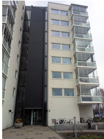
Figure 50. Solar air installation mounted above the entrance of building. Photo: The Author.
