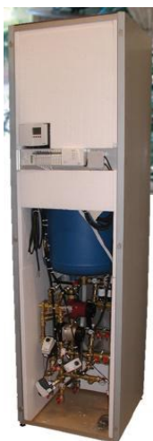
Figure 4.2 Picture and scheme of the district heating storage unit.
