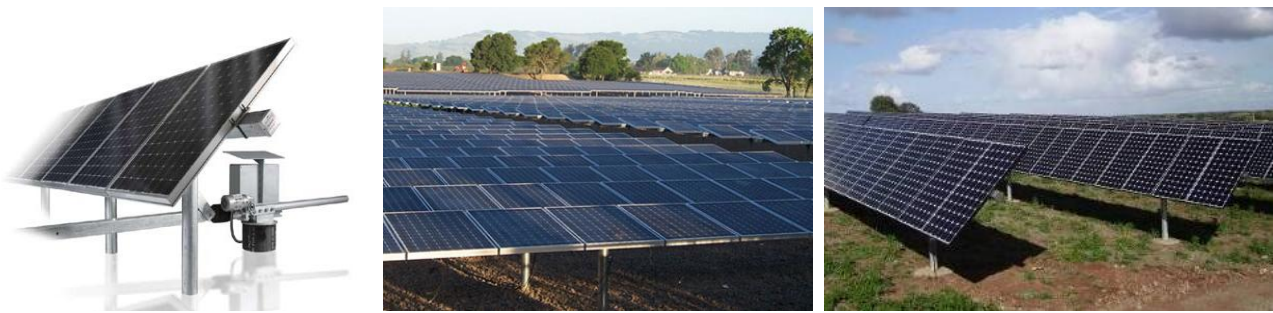
Figure 30: The SunPower T0 horizontal tracker.
