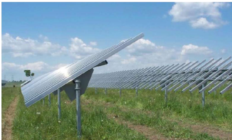
Figure 14: Ground mounting system ready for module installation.
