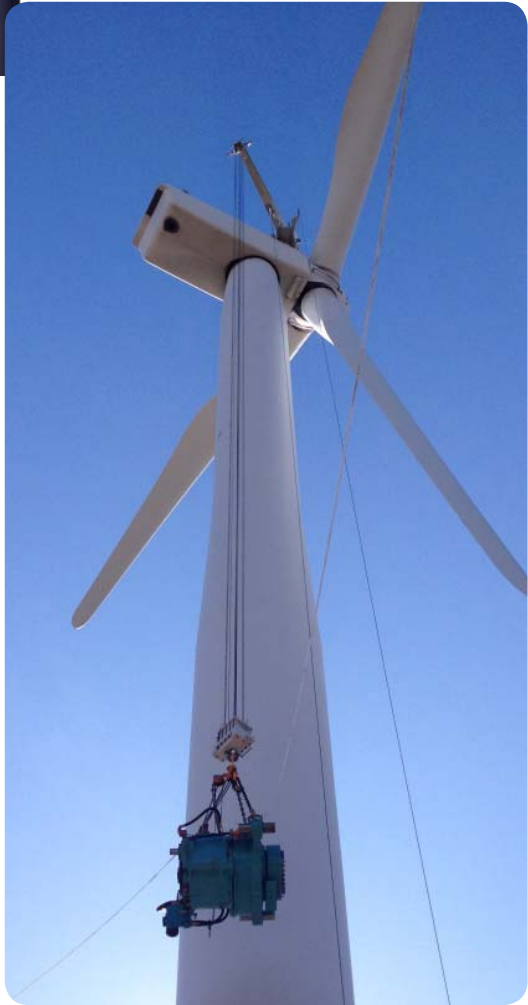
When the cover is removed the gearbox is ready to be changed without use of a mobil crane.
