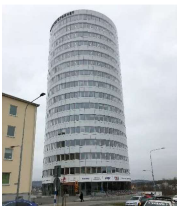
Munksjötårn in Jönköping, Sweden was used for full scale demonstration
