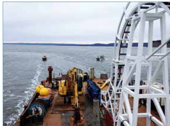
Figure 2 - Cable Laying at the FORCE Site (Source: FORCE)
