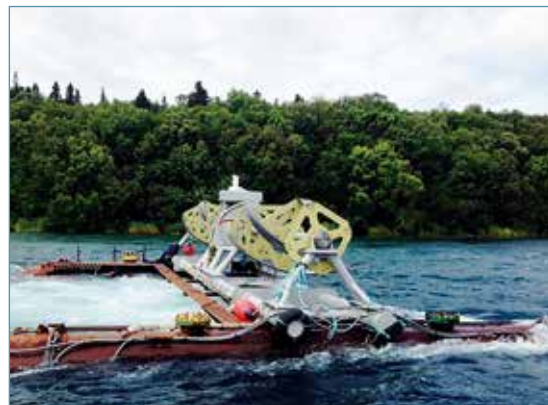
Ocean Renewable Power Company's RivGen turbine prior to being lowered into the Kvichak River in Alaska
