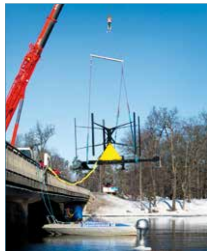
Picture from March 2013 when the marine current energy converter was being deployed in Dalälven river
