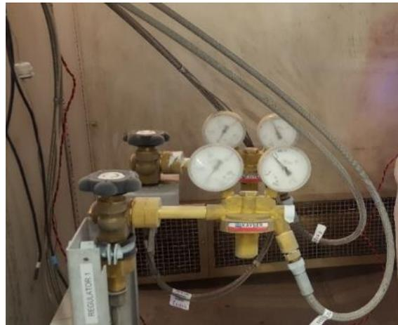
Figure 18 Regulators installed in climate
