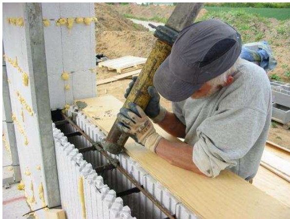
Figure 4: Expanded polystyrene blocks filled with concrete.
