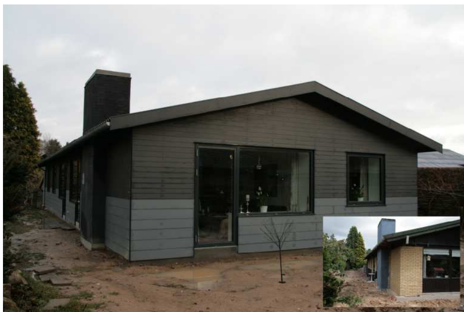
Fig. 1: Photo of the south façade, before and after the energy renovation.
