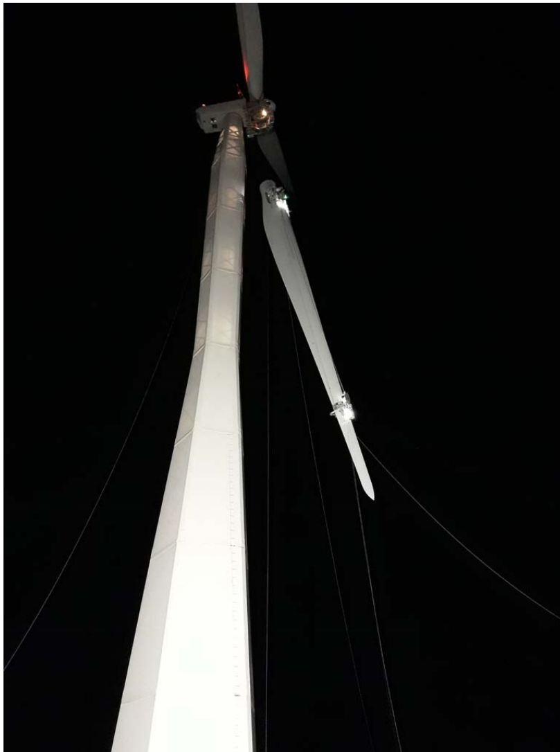
Lowering of the blade from the hub
