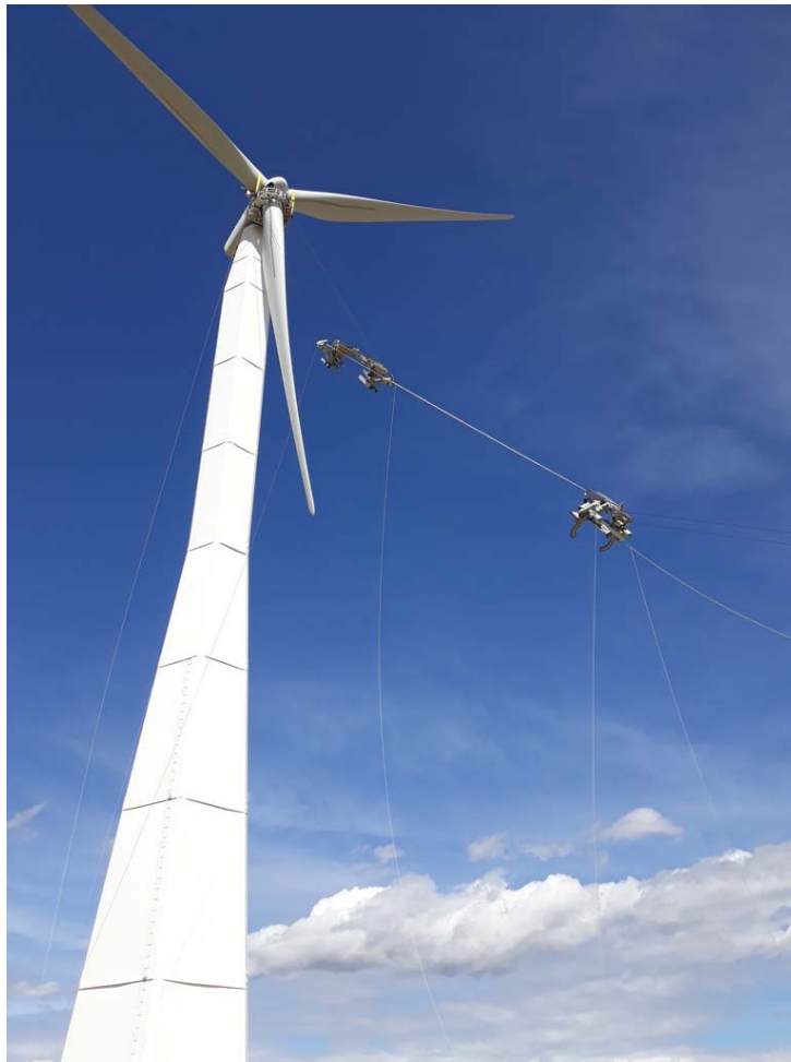
Lifting of the Tip and Root clamp up to the blade
