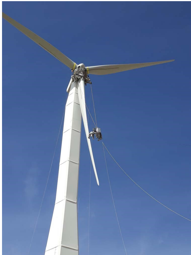
Installation of the Tip and Root clamp on the blade
