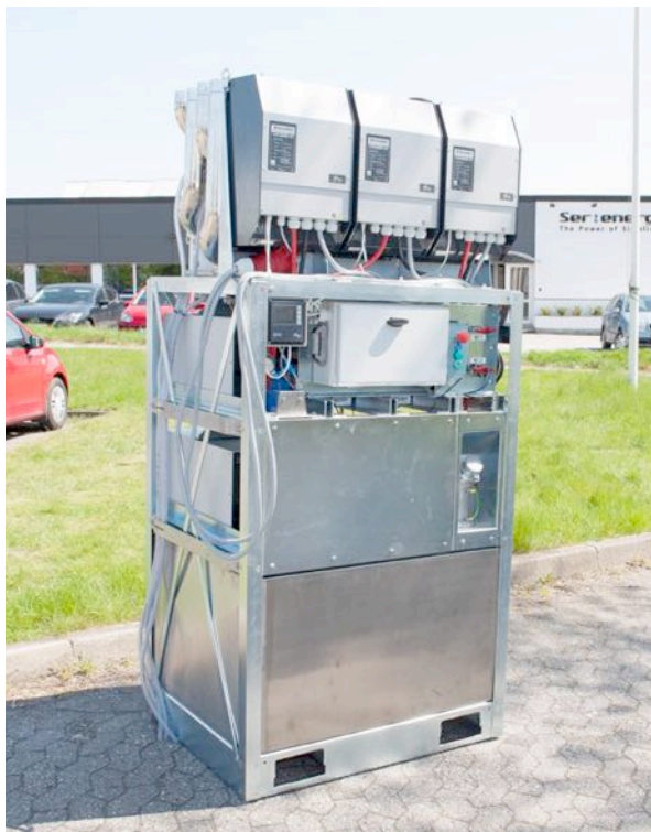
Figure 19 – Per Aarsleff system, view 1
