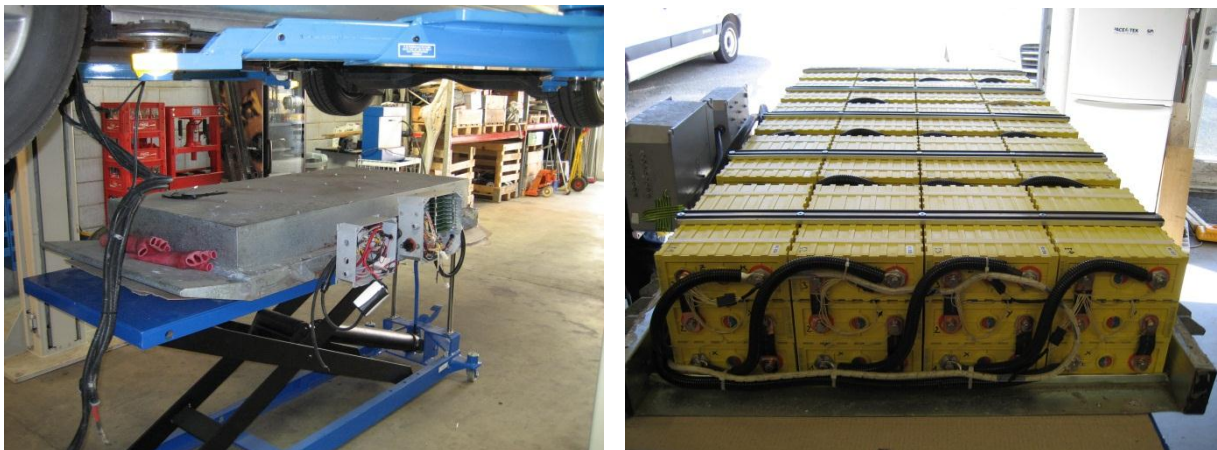
Figure 5 Battery pack dismantled from car. BMS and switching components are placed in the two small boxes on the side. The right picture shows the battery cells inside the pack.
