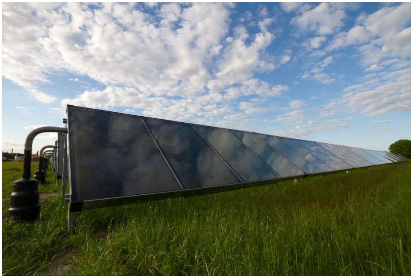
Figure 5.1.1. Row end collector with stanchion
