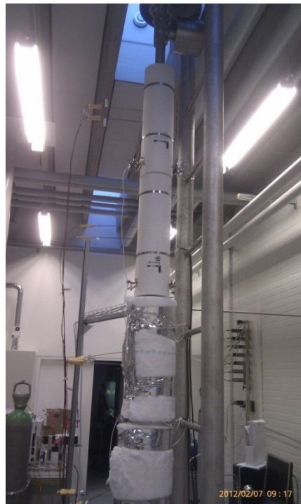
Figure 3: Pilot reactor with visible heating elements
