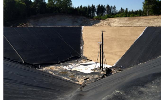
The storage in Dronninglund is situated in an abandoned gravel pit. This made the excavation easy compared to Marstal, where clay caused problems as excavation took place in a rainfull summer.
