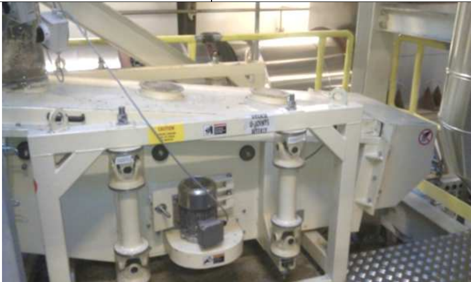
Vibratory Screen Installation for chips cleaning prior to torrefaction.
