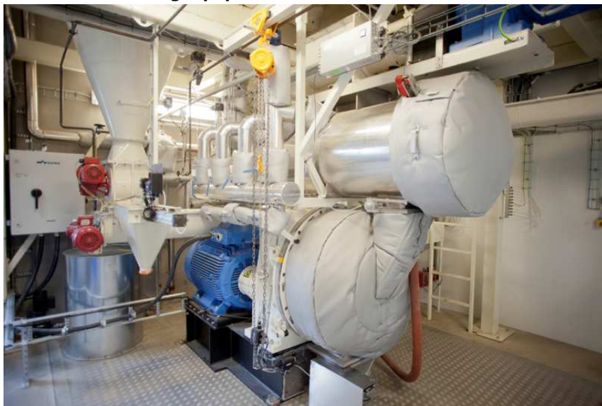
Material pre-conditioning and pellet press installation in the test plant.
